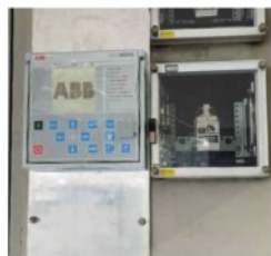
Electromechanical Relays were disconnected from the panel and REF 615 Relays were successfully Retrofitting at Toba Pulp Lestari Site
