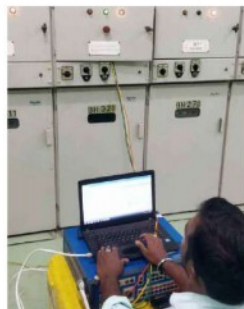
Our Engineer Mr. Ramakrishnan performing the testing of REF 615 Relay using Omicron CMC 356 Test Set after the retrofitting activities at Toba Pulp Lestari Project
