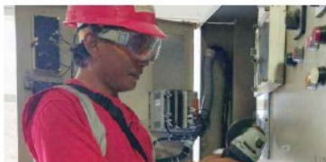
Our Technician Performing the cutting of panel as per dimensions of REF 615 Relay
